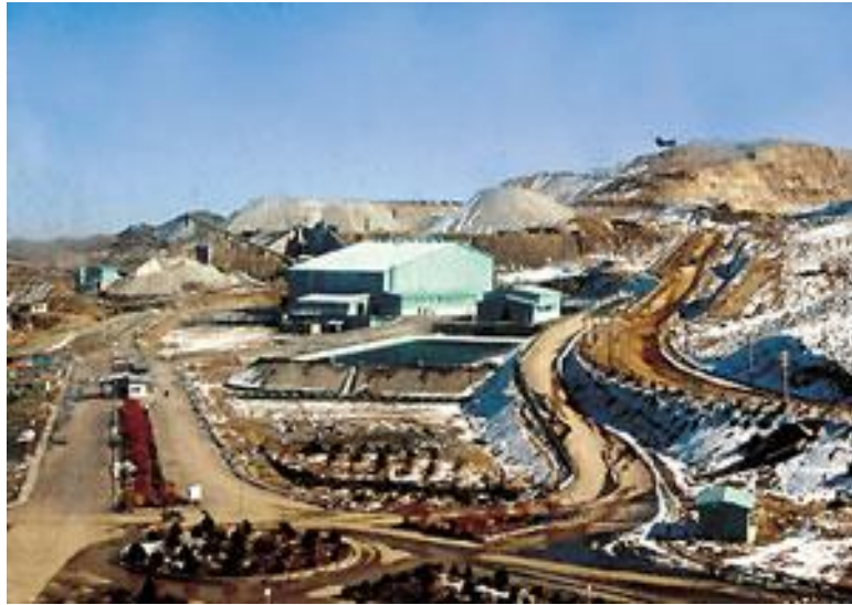
Figure 87. Miduk Copper Complex
